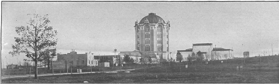
View of The Lewis Publishing Company's plants from the north, University City. The two great plants occupy 8½ acres of beautifully parked grounds.
