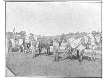
Grading and rolling a street with the mule teams of Alderman Lamb.
